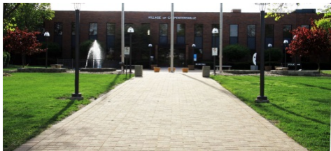
Carpentersville Branch Court
